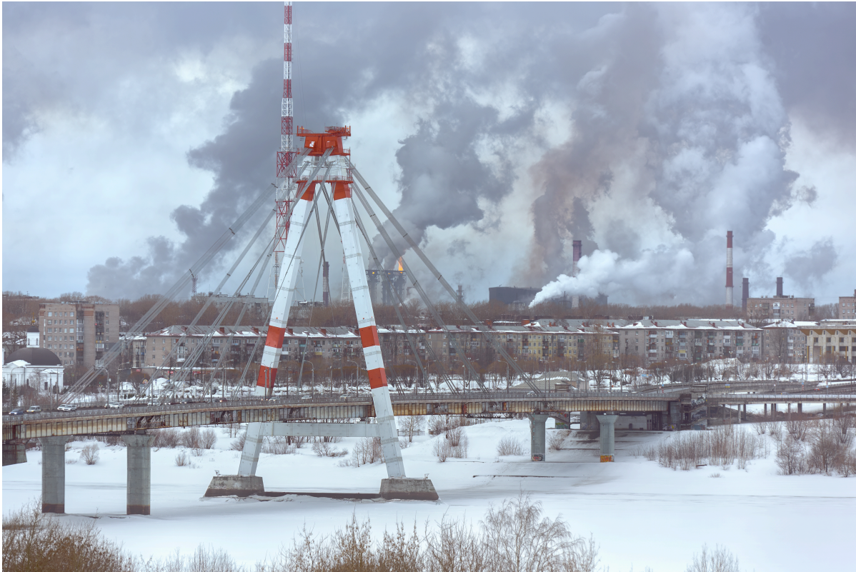
View of the Oktyabrsky Bridge and the factories behind it in the industrial city of Cherepovets, Russia. The output of war-related industries in Russia has increased by over 50 percent compared to antebellum times. © Lexis_Jan on Adobe Stock. All rights reserved.
